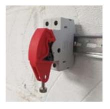
2. Engage the lockout device on the toggle
